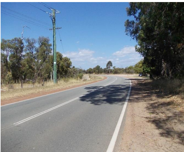
PHOTO 9 Facing east along the road (cleared land).
